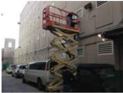
During installation work at Orleans Parish Prison.
